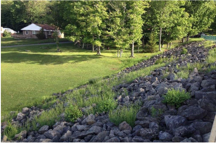
Downstream slope north of the primary spillway.
