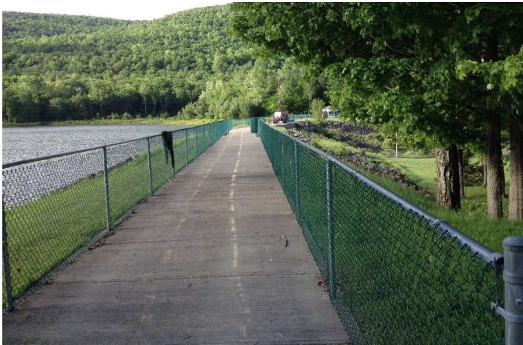
Dam crest – concrete walkway.
